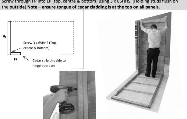
When screwing the four corners together please make sure the studs are flush on the outside (not the inside) as per image below.
