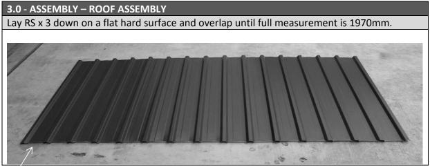
Bent up edge goes at the back of the shed.
