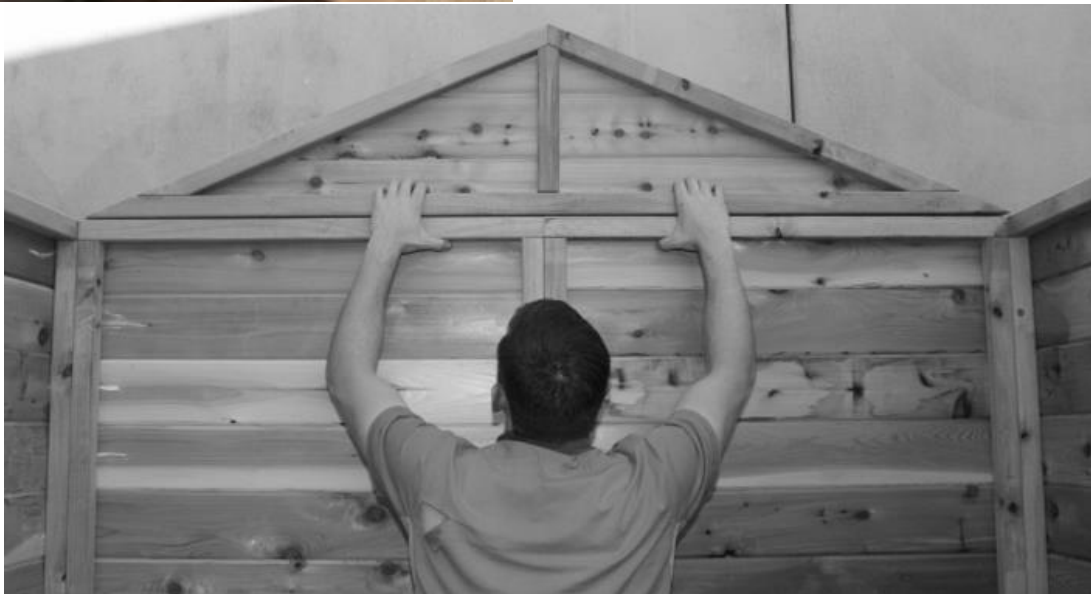
Ensure groove slots into tongue
