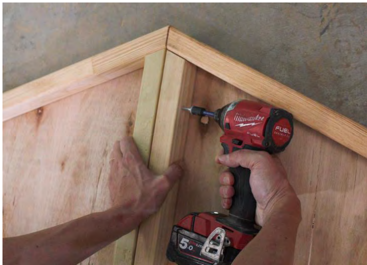
Hold flush at the bottom and fasten together with 2x 65HHS
