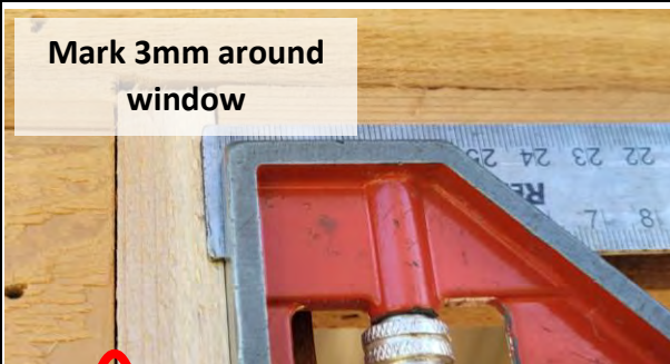
Measure, mark and cut side strips to size
