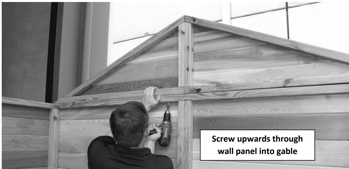
Ensure groove slots into tongue
