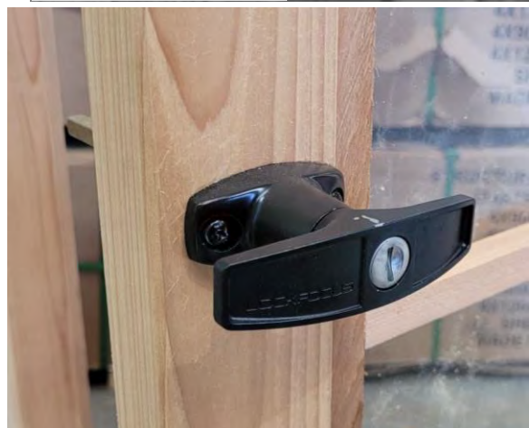
Drill 6mm holes and fasten t-handle to door with bolts, nuts, and washers.
