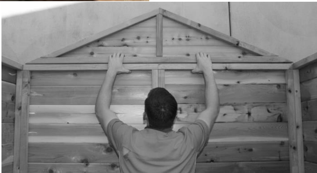
Ensure groove slots into tongue
