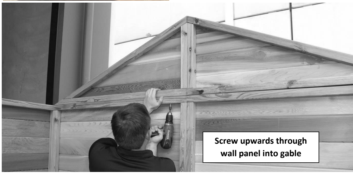
Ensure groove slots into tongue
