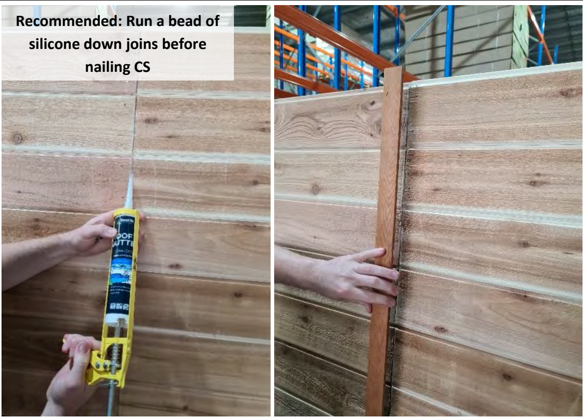
Nail 6x 40N evenly spaced along CS
