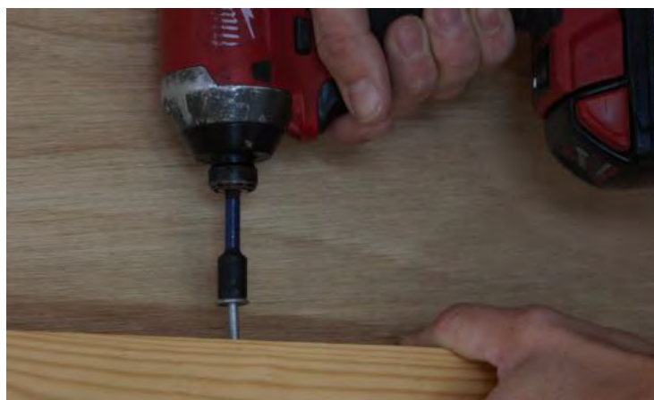
Screw 3x 65HHS down through gable into door head.
